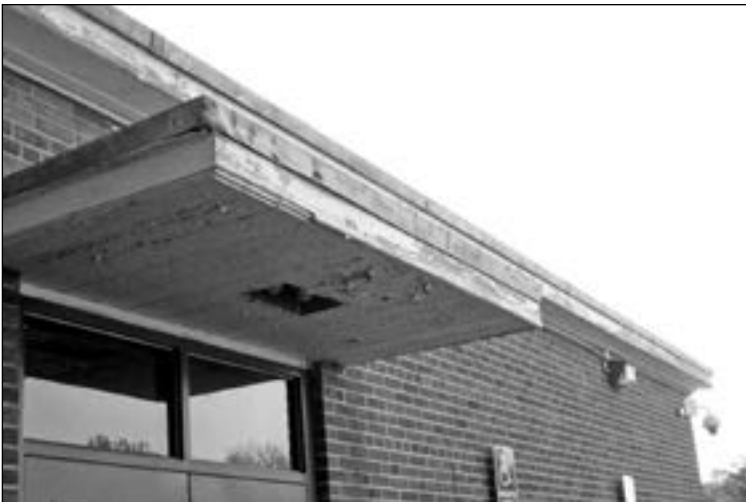
Fascia board will be replaced at Parkville .
